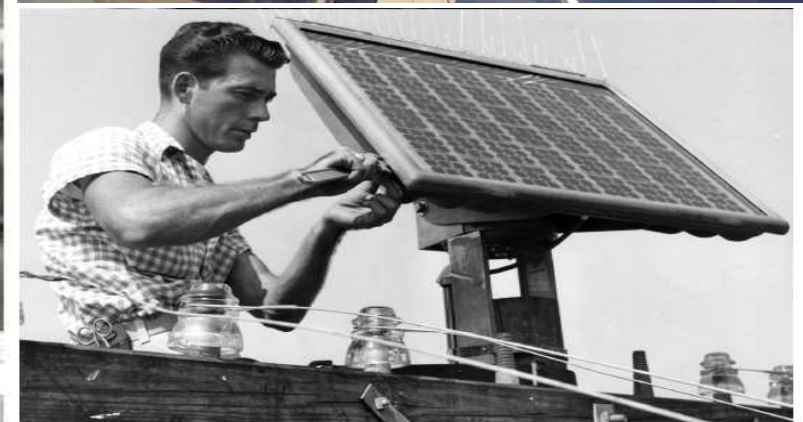
Fig. 3. Americus, Georgia module used to power telephone repeater, being lab assembled, showing submodule of cells encased in oil (top) and deployed in southwest U.S. location (bottom).
